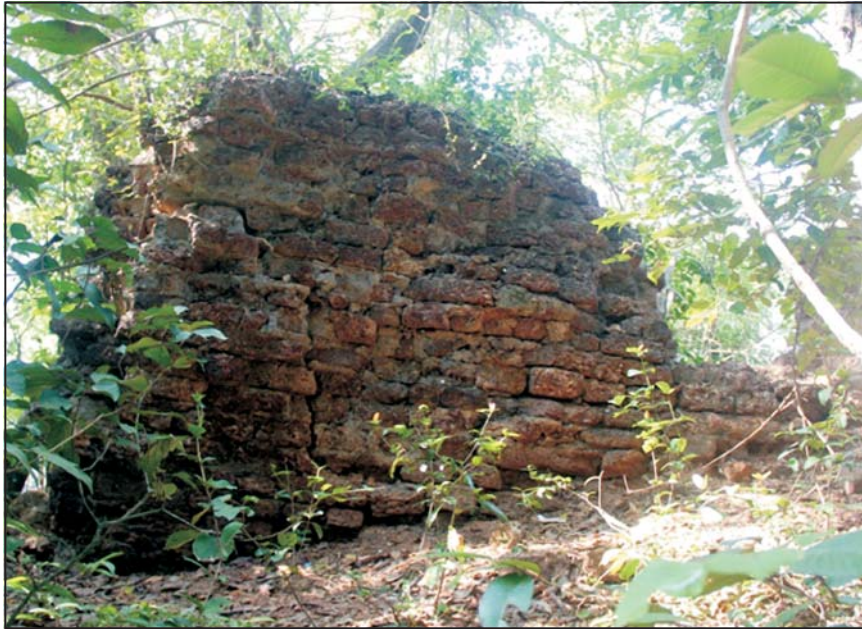
Southern Wall of the Dharmadam Fort
